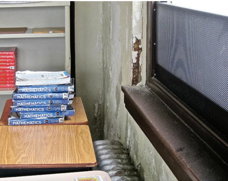
(Above) A 3rd-floor classroom with damaged lead paint and plaster, long-term and unattended water intrusion, and dust/debris on surfaces — a major asthma trigger. The black security screen on the inside of the window was installed as an interim solution after a substitute teacher lost three of her fingers when a window crashed down on them.
